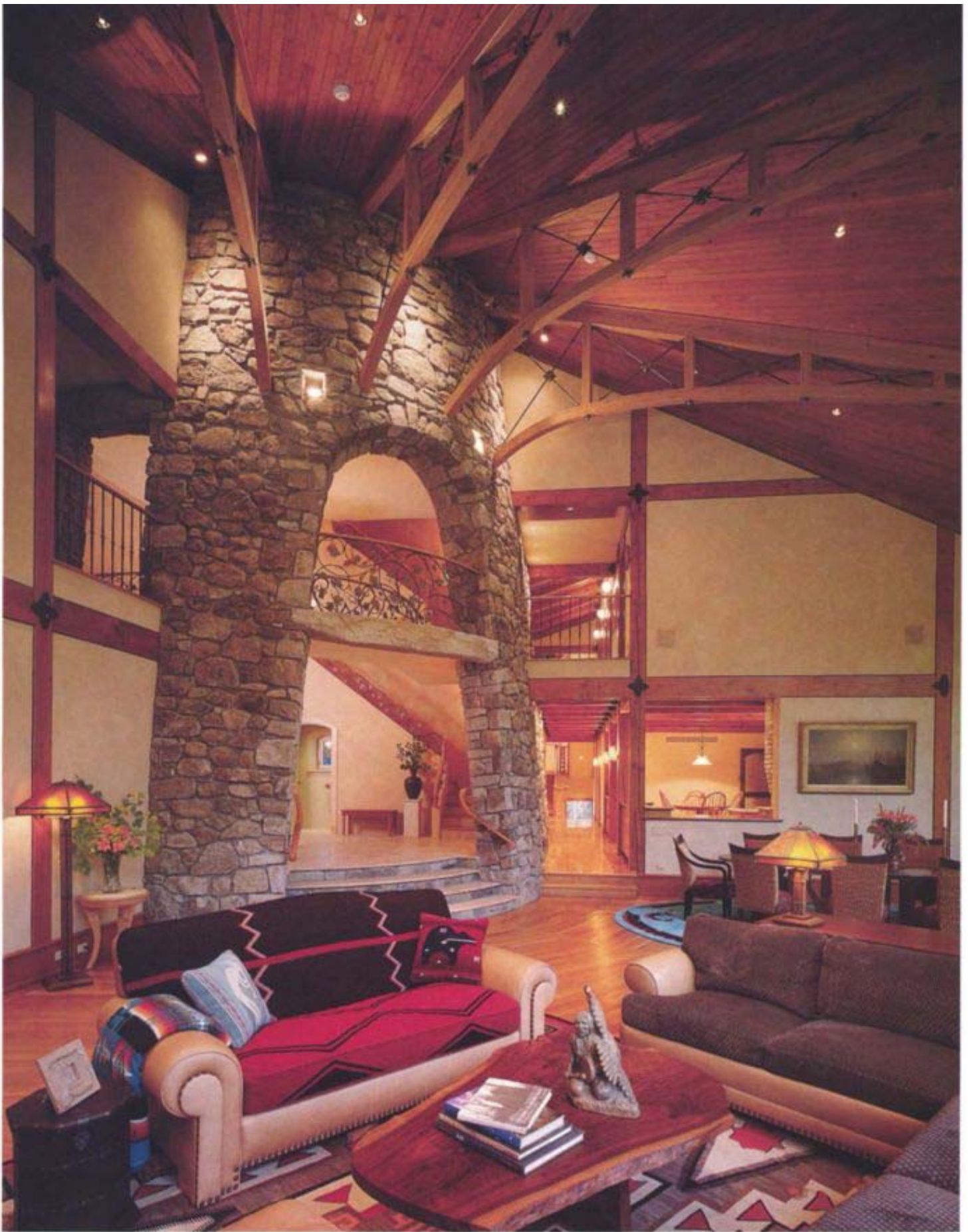
Great room benefits from the strength of soaring glulam trusses. By concealing the glulams' top chords in the ceiling, the architect managed to design trusses that were strong enough to hold a large copper roof, yet appear as light as a Japanese umbrella. The tower's granite, assembled by Mario Gregorio of Cold Spring, New York, came from the site. Photo by Chris Lovi.
